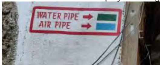
Color Coding for Tunnel air / Water pipeline.
