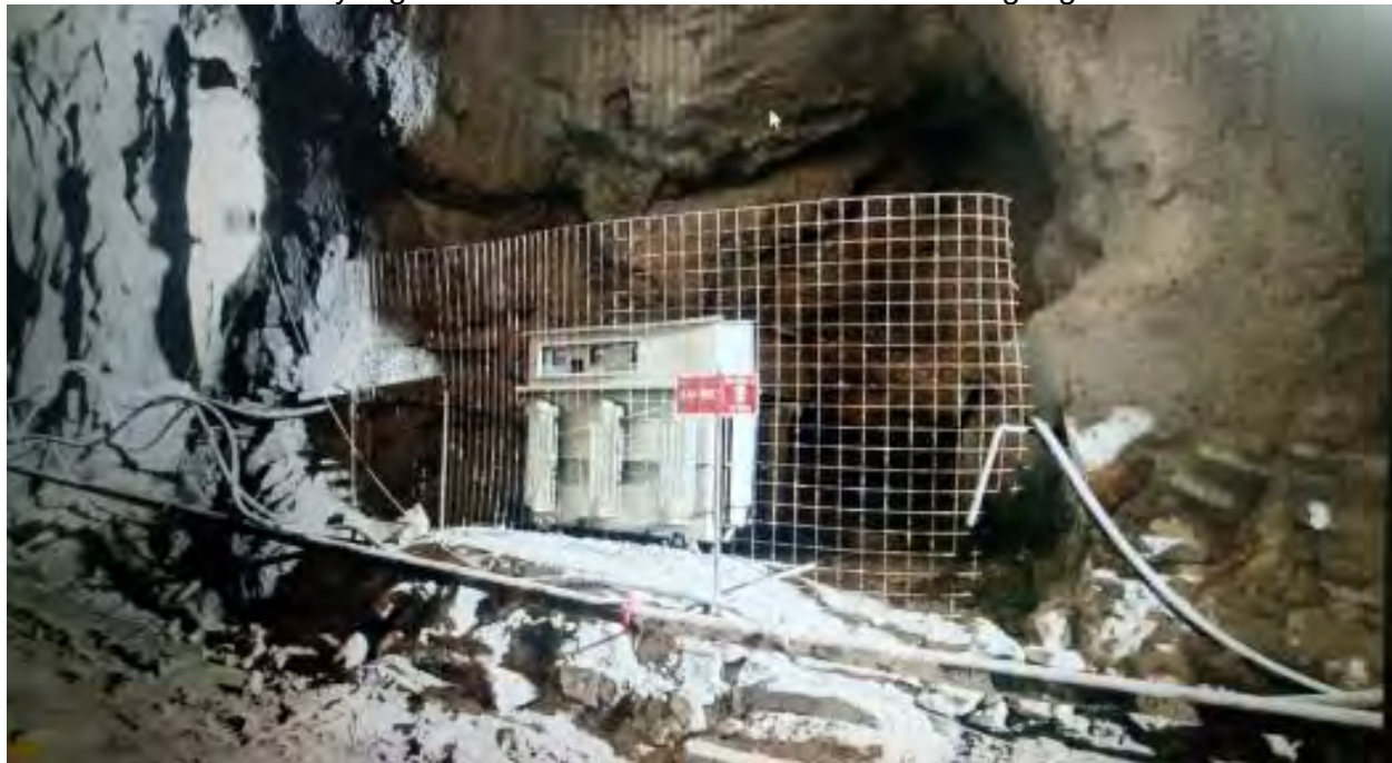
Fancying arrangement for High voltage Electrical equipment at Underground
