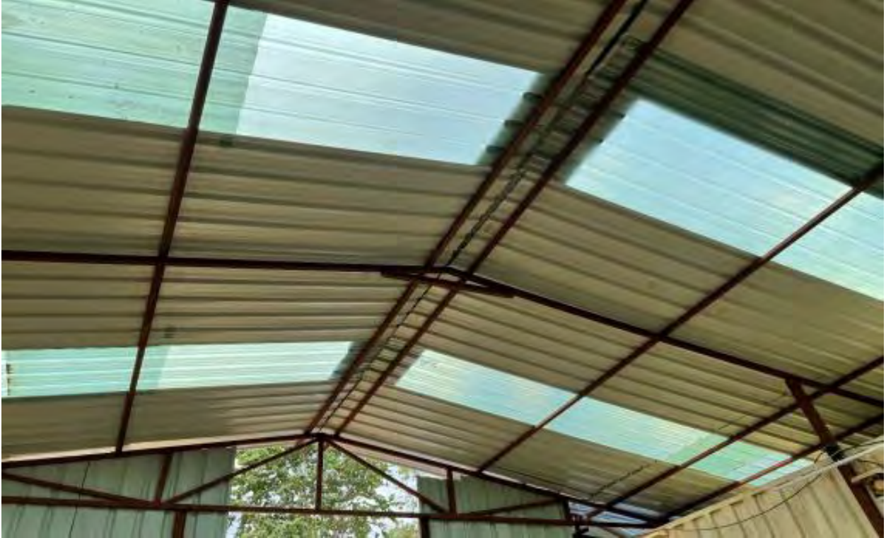
Using transparent sheet in store and other sheds to reduce electricity consumption.
