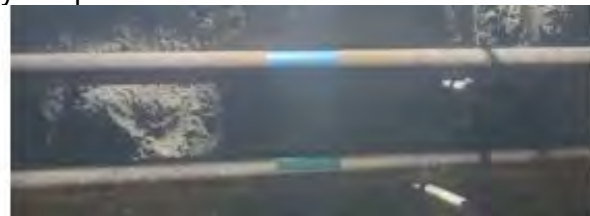
Color Coding for Tunnel air / Water pipeline.
