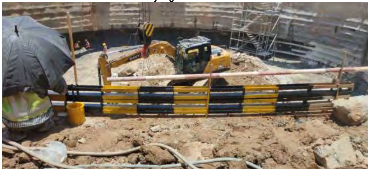
Hard edge protection for Surge Shaft deep excavation
