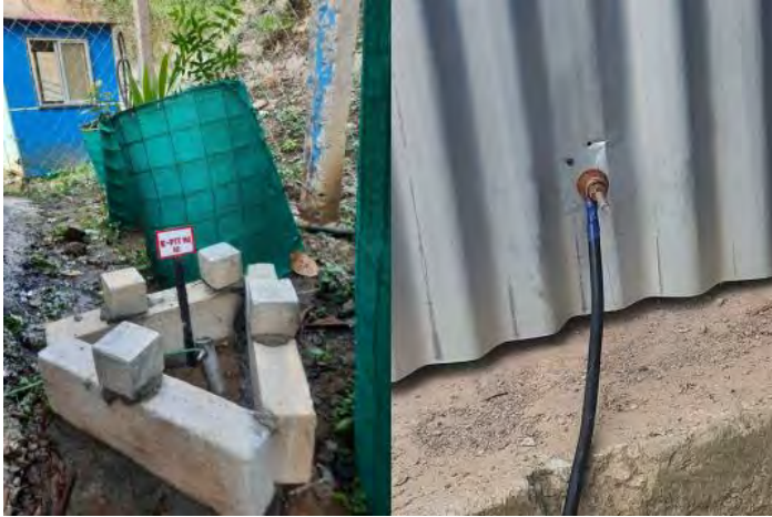
Earthing pit for Metal Office Cabin
