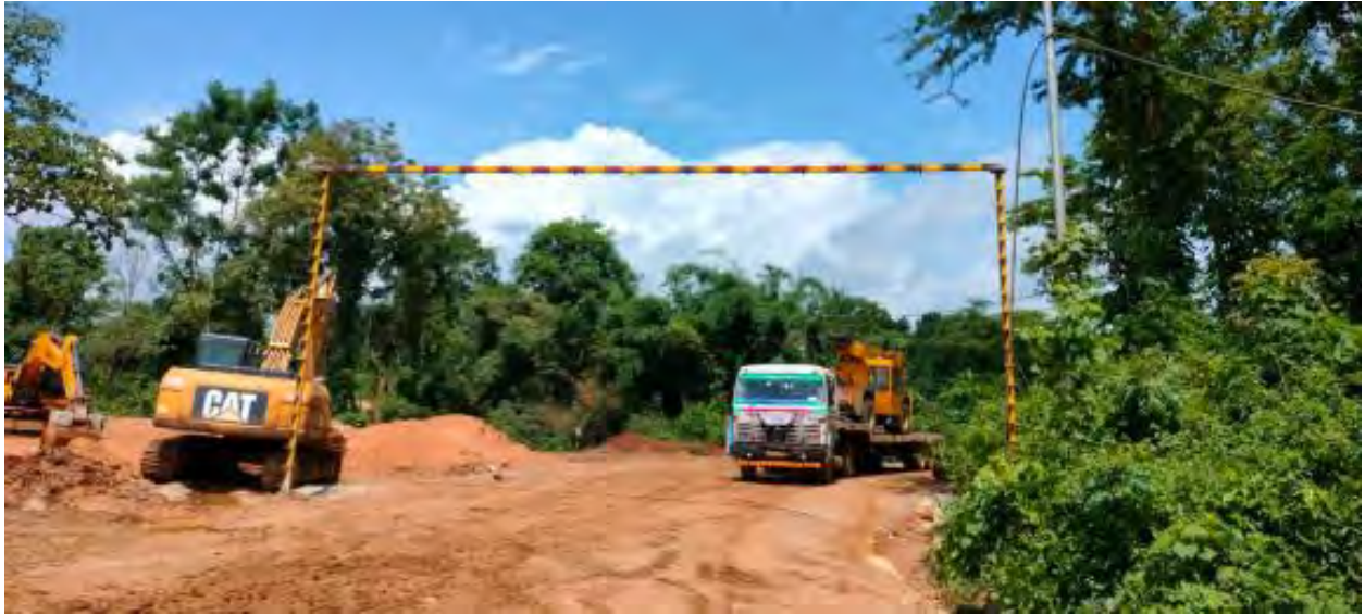
Goal post for overhead electrical line
