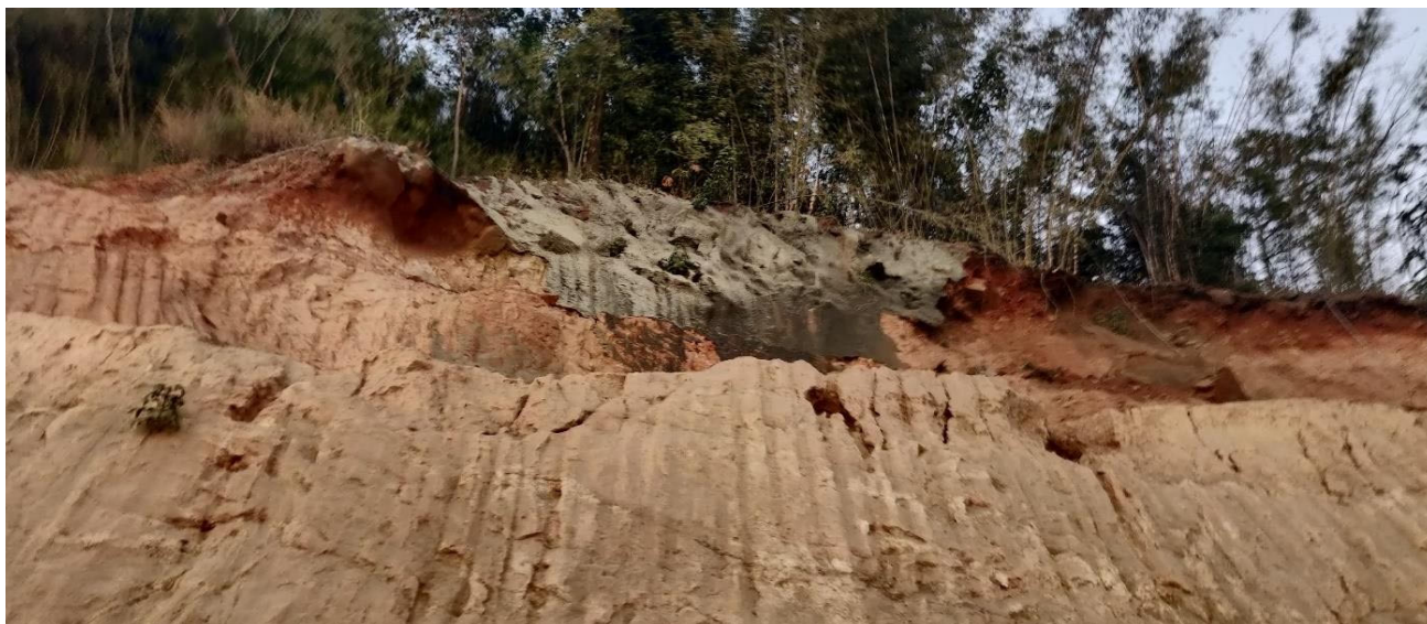
Soil Erosion at Right Bank of Dam Site
