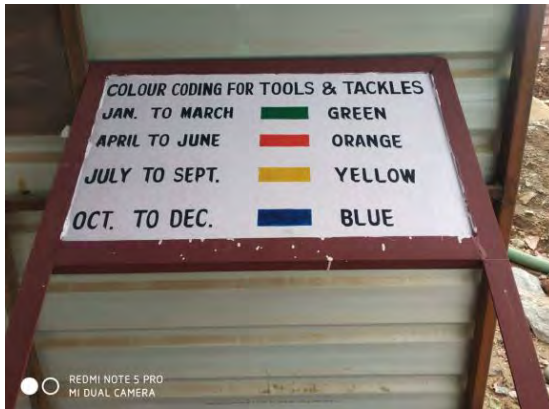
Lifting Tools and tackles color coding system
