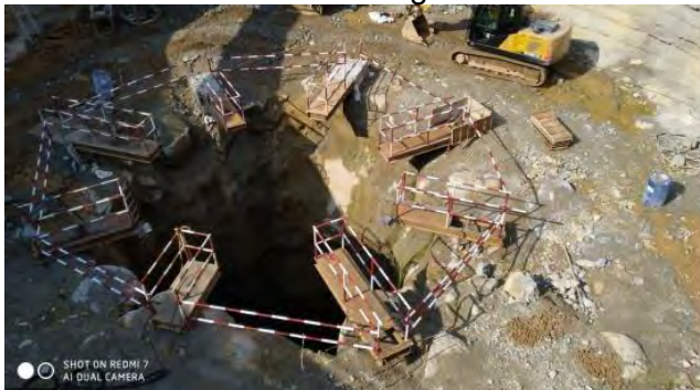
Hard Barricading for Raiser Shaft
